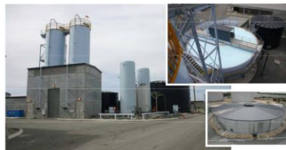
Perth Seawater Desalination Plant Potabilisation System and Drinking Water Storage Tank
