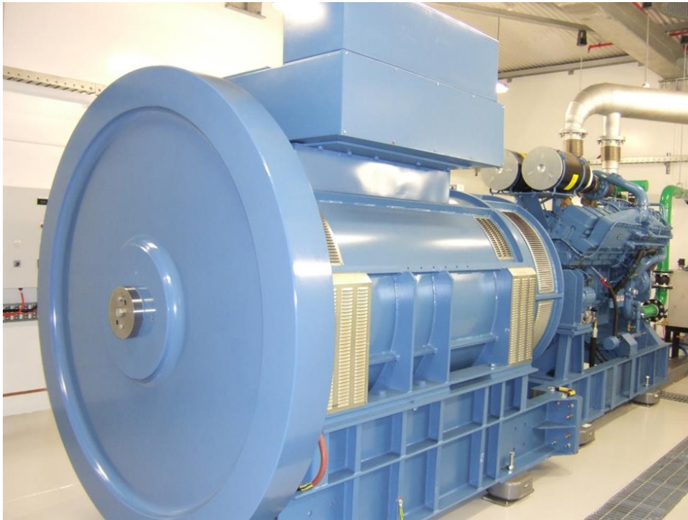
King Island flywheel – supports system without diesel generation Consumes spilled renewables to operate Also an instant start diesel generator to provide firm capacity
