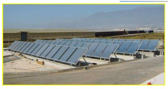
$$A_{r} = \frac{Q_{UV} V_{t}}{T_{s} \overline{UV_{G}}} = \frac{12 x 10^{3} x 1875 x 10^{3}}{3000 x 3600 x 18.6} \left[ \frac{J L^{-1} L}{s W m^{-2}} \right] = 112 m^{2}$$
