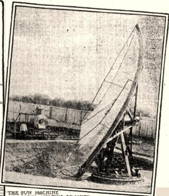
THE SUN MACHINE AT WORK MELTING GRANITE.
