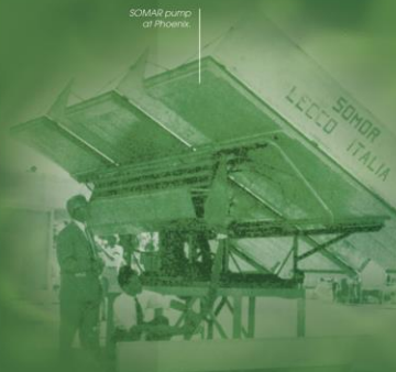
SOMAR pumps at Phoenix.
