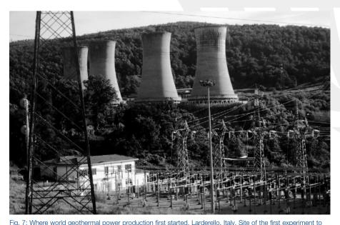
Fig. 7: where word geothermal power production first started, Lardereilo, italy. Site of the first experiment to use geothermal steam to produce electricity, on July 15, 1904, then site of the world's first geothermal powerplant, 250 kW<sub>e</sub>, in 1914. Larderello, located on the hottest geothermal spot in all of Europe, today produces about 400 MW net of geothermal electric power. *Photograph by Dr. Donald Aitken*
