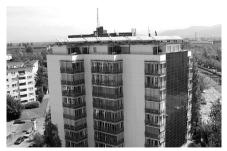
Fig. 16b: A multifamily building in Freiburg, Germany, using the roof for solar water heating, and the south wall for solar electric energy production.
