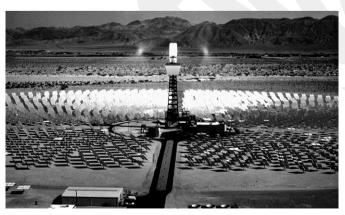
Fig. 14b: Solar I, the 10MW "power tower" in southern California. Source Fig. 14a: NREL Source Fig. 14b: U.S.D.O.E.
