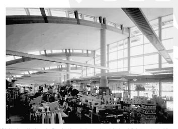
Fig. 12a, b: The Real Goods Solar Living Center, a retail store in Hopland, California, USA (designed by Van der Ryn Architects). A complete "bioclimatic" design, the building features passive solar heating, daylighting, natural ventilation and cooling, PV electricity and native landscaping. Energy savings compared to a conventional design in the Hopland climate are 90 %. In-store sales are 50 % higher than projected because the interior daylighting and comfort are so good.
