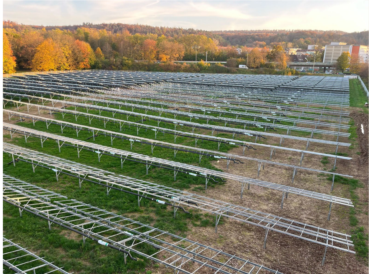
Collector field under construction, as seen from the storage facility
